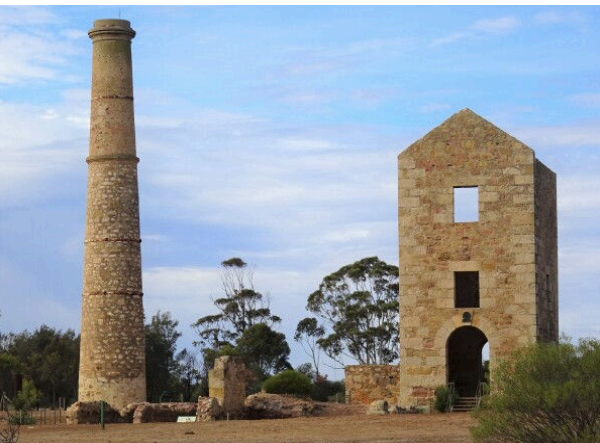
Cornish style enginehouse and round chimney combination
