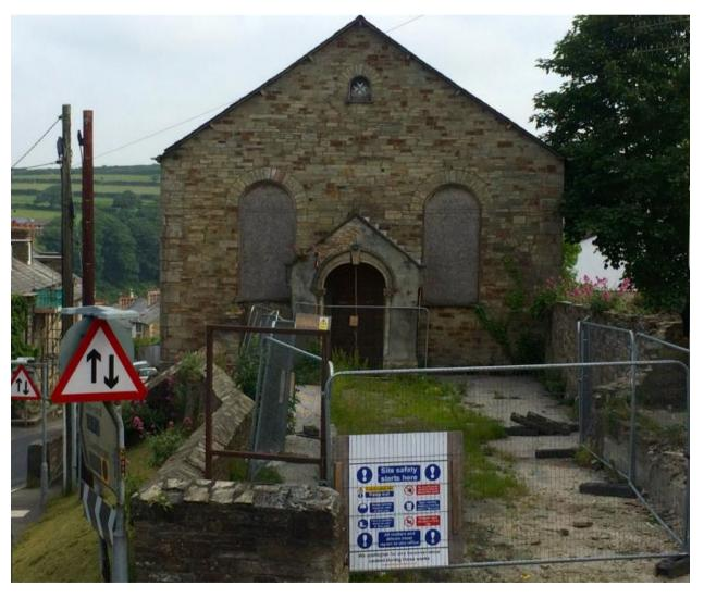
High on our list of concerns, this former chapel is not listed, is in a conservation area and in a very poor condition. A recent enforcement case was assigned to Cornwall Council Building Control because of falling slates and serious cracks in the fabric.
