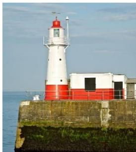
A hole extends through the floor of the hut down into the harbour wall forming a chamber with an inlet pipe connected to the sea. Equipment in the shed is linked to a float in the chamber and records the rise and fall of the tides. The chamber layout eliminates most of the wave movement.
