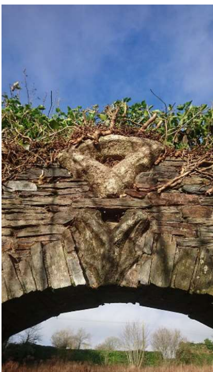
Above – historic wall structure with inserted medieval stone tracery.
