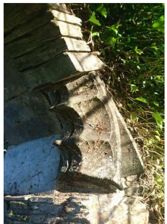
Above – historic wall structure with inserted medieval stone tracery.
