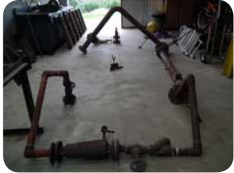
into water. Due to the lack of drainage in several places, a large quantity of standing condensate was causing water hammer and corrosion in the pipe. Finally, following comments by both the Boiler Engineer and the Inspector that the design would encourage pulsing, the decision was taken by the National Trust to replace the pipe work during the winter maintenance of 2018/19.
