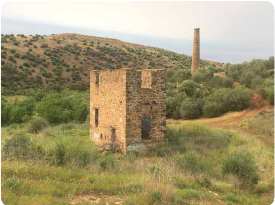
Fig. 4: Front view of the all-enclosed engine house and separate stack at Worthing Mine, showing masonry mounting block alongside the crankshaft opening. Middle Gully (Engine) shaft lies just out of view to the bottom right.
