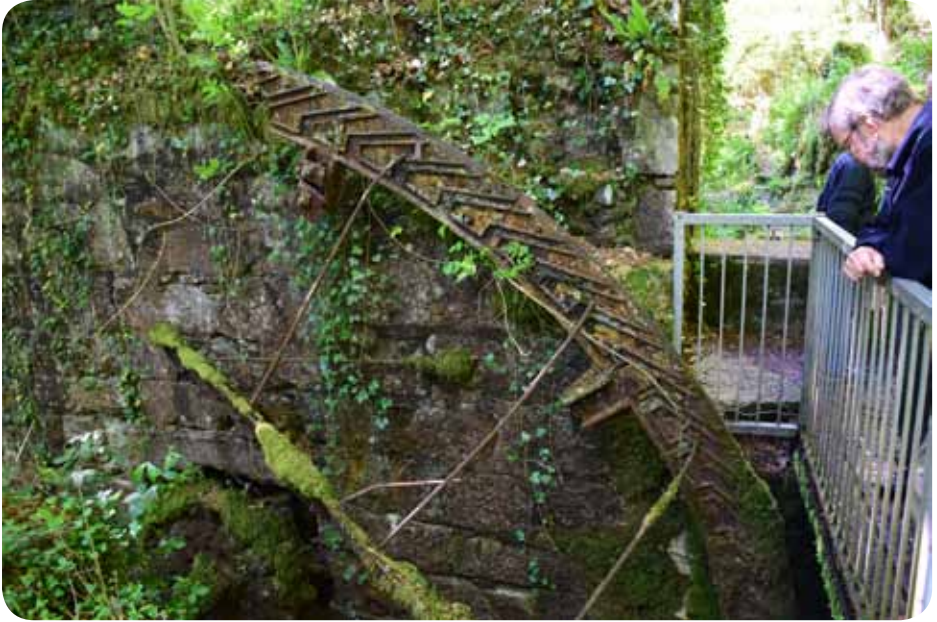
The remains of the overshoot waterwheel which sat between two mills massively constructed of granite blocks. The remnant gearing seen below was in a room below the mill bed, to reduce the risk of explosion. The roof of these mills was flimsy so any such explosion was directed to the heavens.
