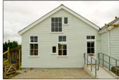
above: The exterior of King Edward Mine's new Winder and Compressor house, a replacement following the 1957 fire. Construction follows closely the original surviving buildings most of which are Listed Grade II\*.
