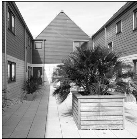
above: inside the housing court on the top levels at Maritime House, Falmouth
