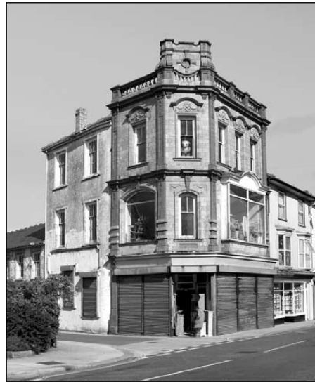
An imposing edifice to improve his town's standing [Commercial Street, Camborne]
